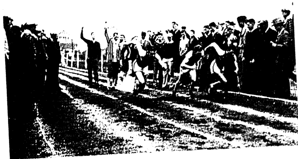
Bridges and Gates off to a quick start
